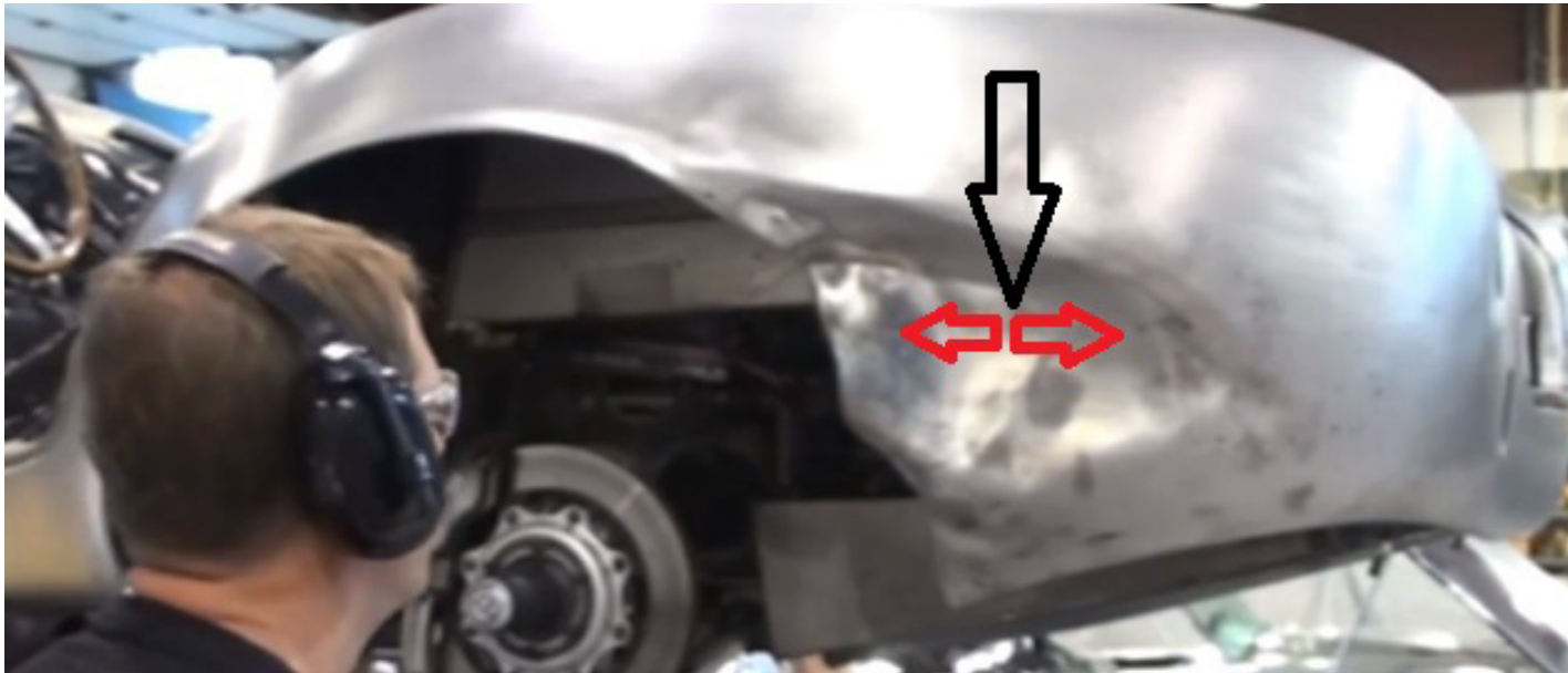
Work outward from the deepest part
